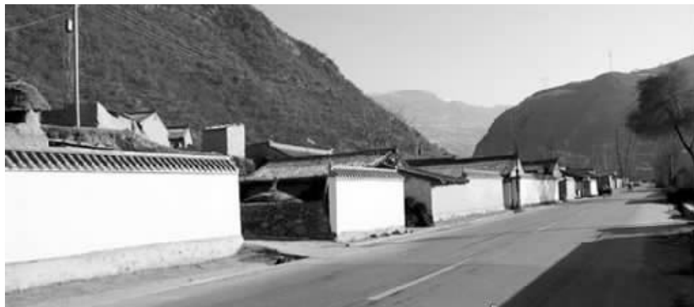
甘肃漳县殪虎桥乡东桥村,一排已经粉刷过的“遮羞墙”
