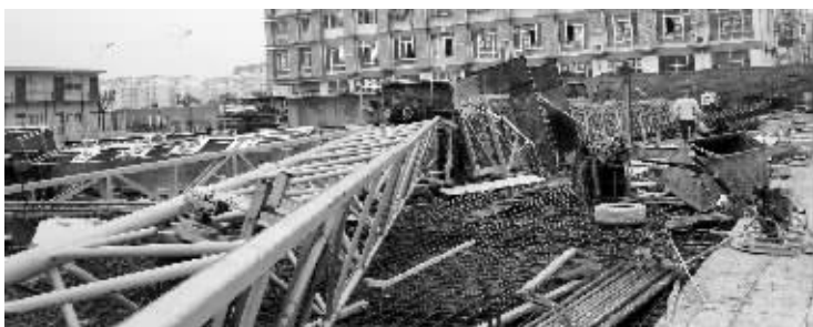
倒塌的塔吊
