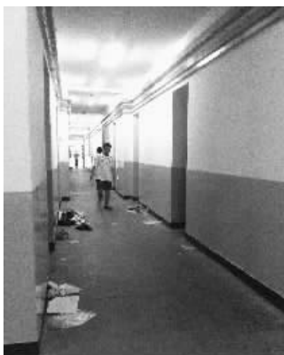
宿舍走廊刚漆过
