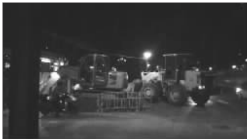
清扬路夜间仍在施工 匡笠 摄
