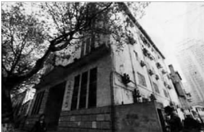
▶大楼被拆之前的模样
